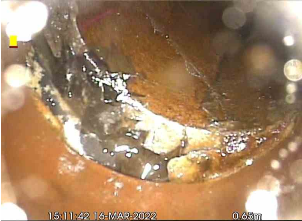
15:11:42 16-MAR-2022 0.65m G4X_796243bf-c306-4f28-8d52-dd3f4df6e185_20220328_111658_902.jpg, 00:00:07, 0.65 m Joint displaced, medium
