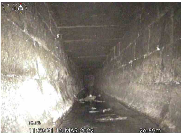
FW1X_69f4a7af-3fb3-41be-b891-e3a4ea12a504_20220325_114750_905.jpg, 00:06:33, 26.89 m Settled deposits, fine, 10% cross-sectional area loss, start
